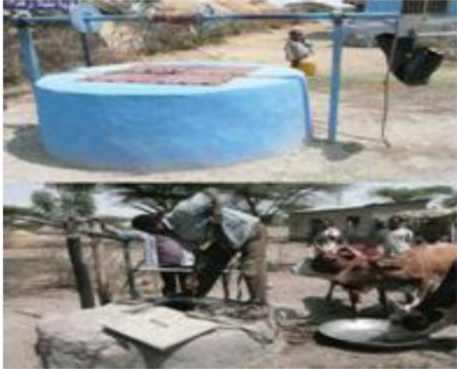
Figure 7.5: Two wells with concrete protection.
