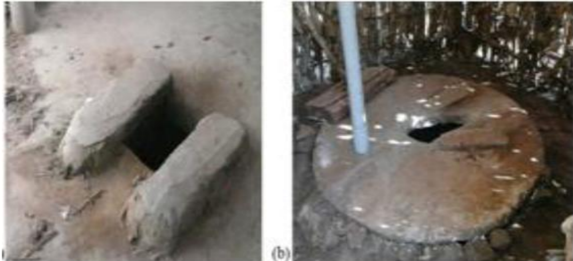
Figure 7.2: (a) Slab with raised footrest in a pit latrine. (b) Round cement slab
